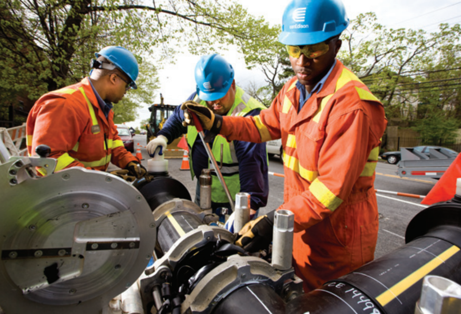
Gas workers in the Bronx fuse new pipe.
