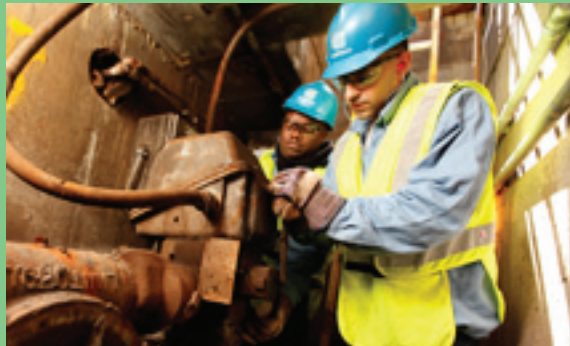
Steam workers perform maintenance work.
